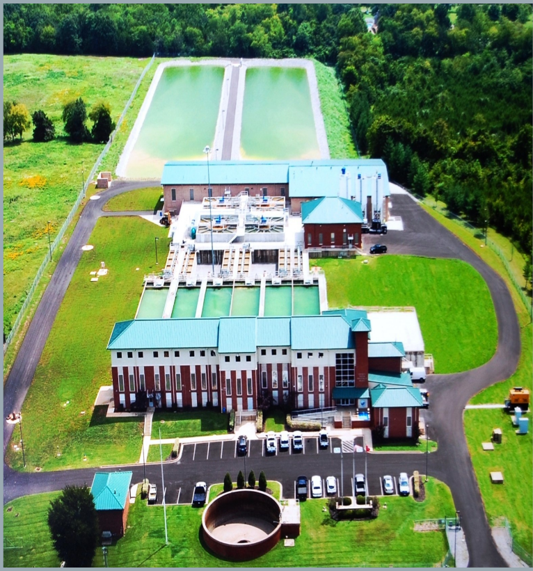
Town of Smyrna Water Treatment Plant
